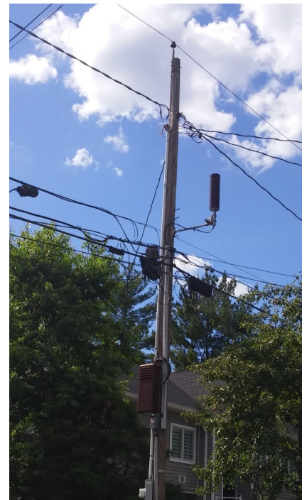
Typical Antenna Installation
